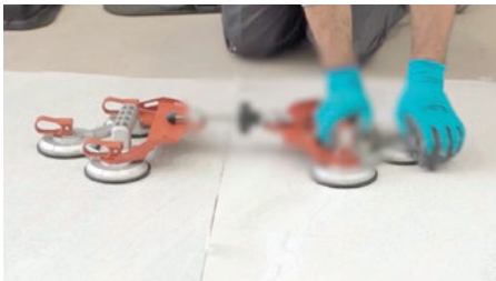
Dispositivo accosta-lastre / Special device for the plate's pulling-over
